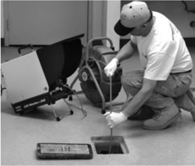
Figure 28 – Proper Cable Push
