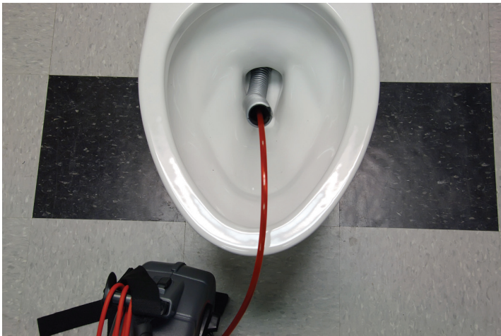
Figure 24 – Using the Flexible Guide Tube
