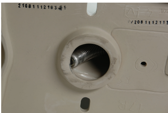
Figure 17 – Camera Head Blocked in Turn
