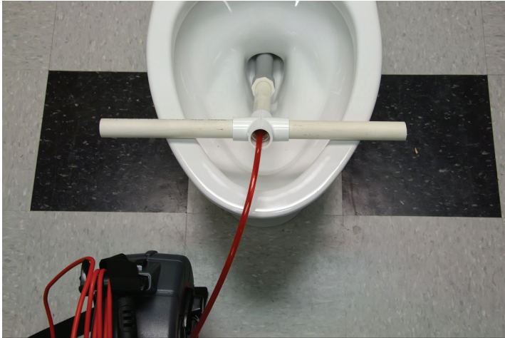
Figure 23 – Using a PVC Guide Tube
